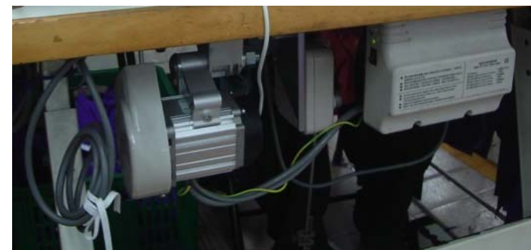
Proper maintained motor
